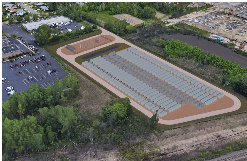
Project above is 150MW/300MWh (2hrs duration) on 5 acres
